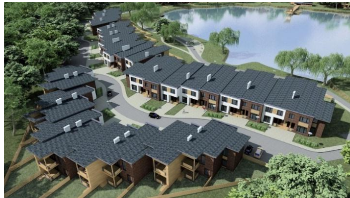
Fig.4. Innovative modular residential buildings
